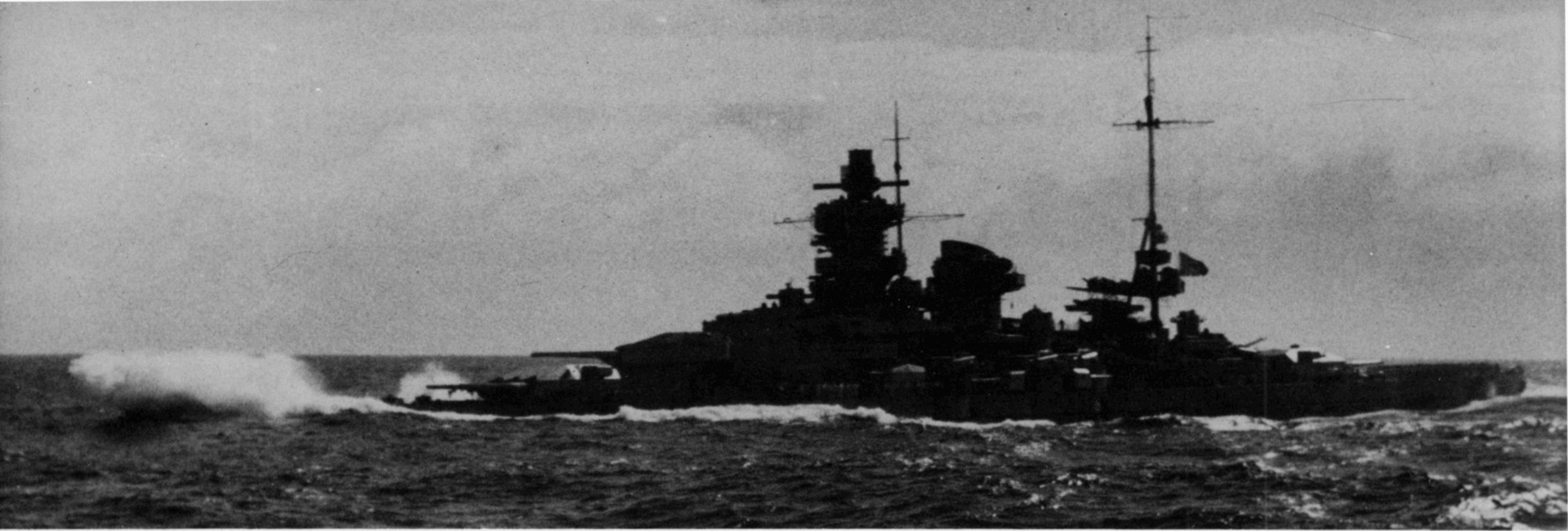
In the swells of the Atlantic. This picture was taken during Operation "Berlin" (January to March 1941). Here the poor trimming characteristics of the SCHARNHORST (the same was true of the sister ship GNEISENAU) became especially clear. As a result of the great weight forward, the bow took a great deal of water; rebuilding did very little to change it. The forward turret was always bothered by it.
