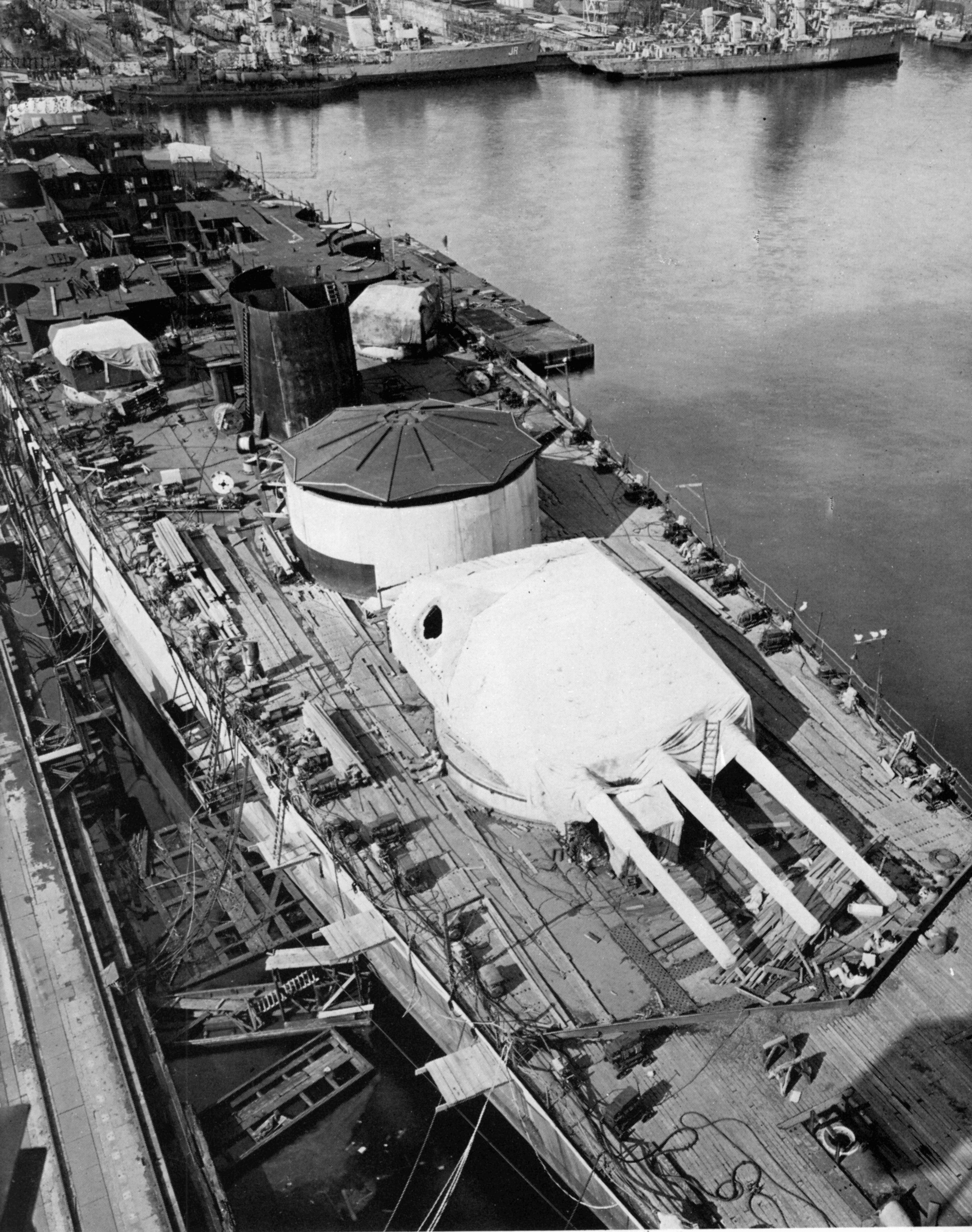
This picture was taken during the work of fitting out the ship, presumably in 1937. The "Anton" turret is already mounted. Behind the barbette of the "Bruno" turret, the raw structure of the armored bridge can be seen.
