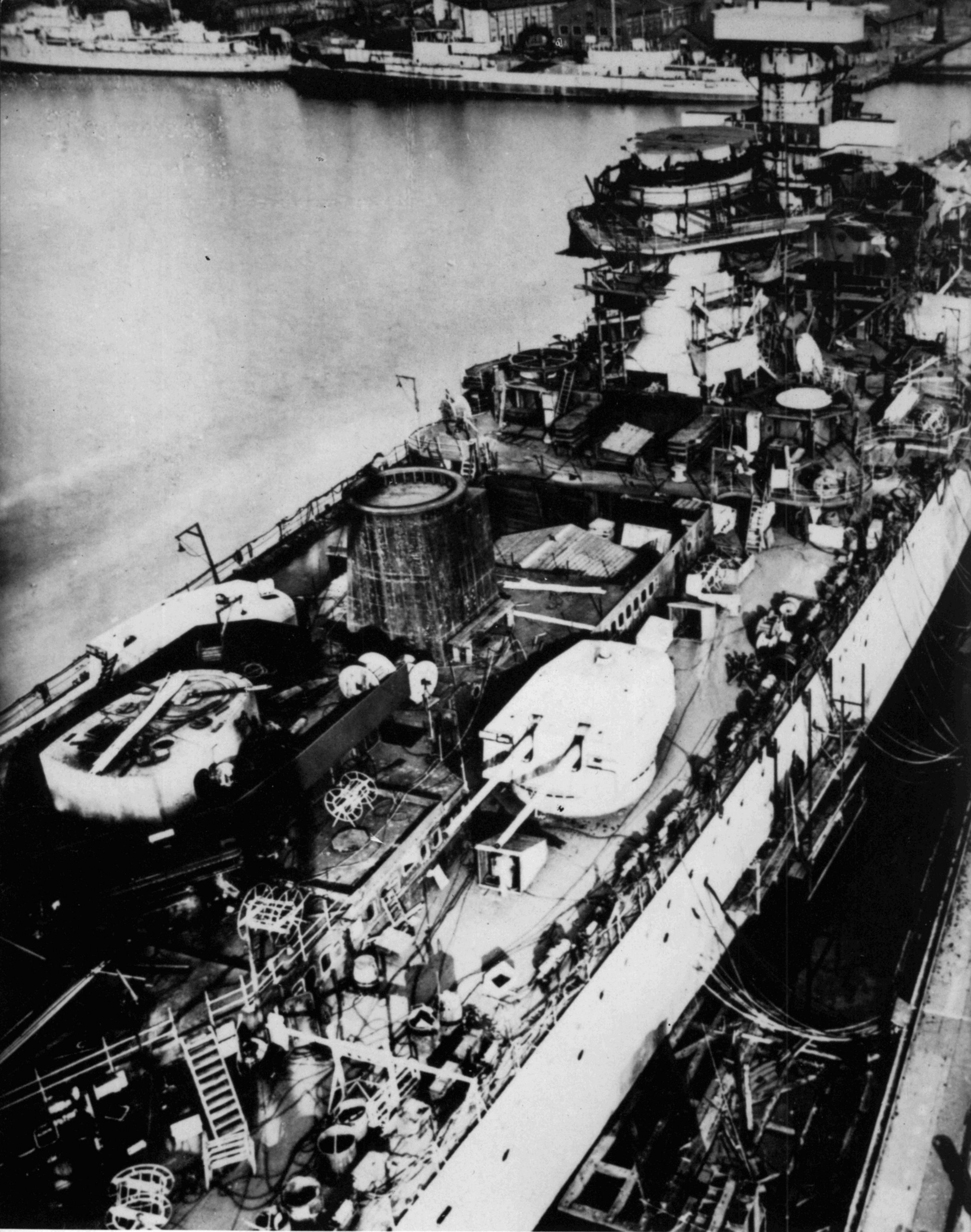
This picture was probably taken toward the end of 1937 — maybe even later. Here the superstructures have been erected and the 15-cm twin turrets installed. Behind the already installed catapult tower the shafts for installing the machines and boiler can be seen, and are not yet closed off.
